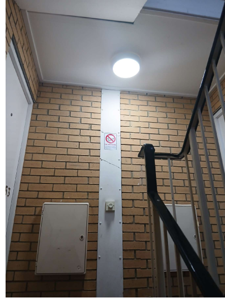
Lighting (Standard and Emergency Lights)
